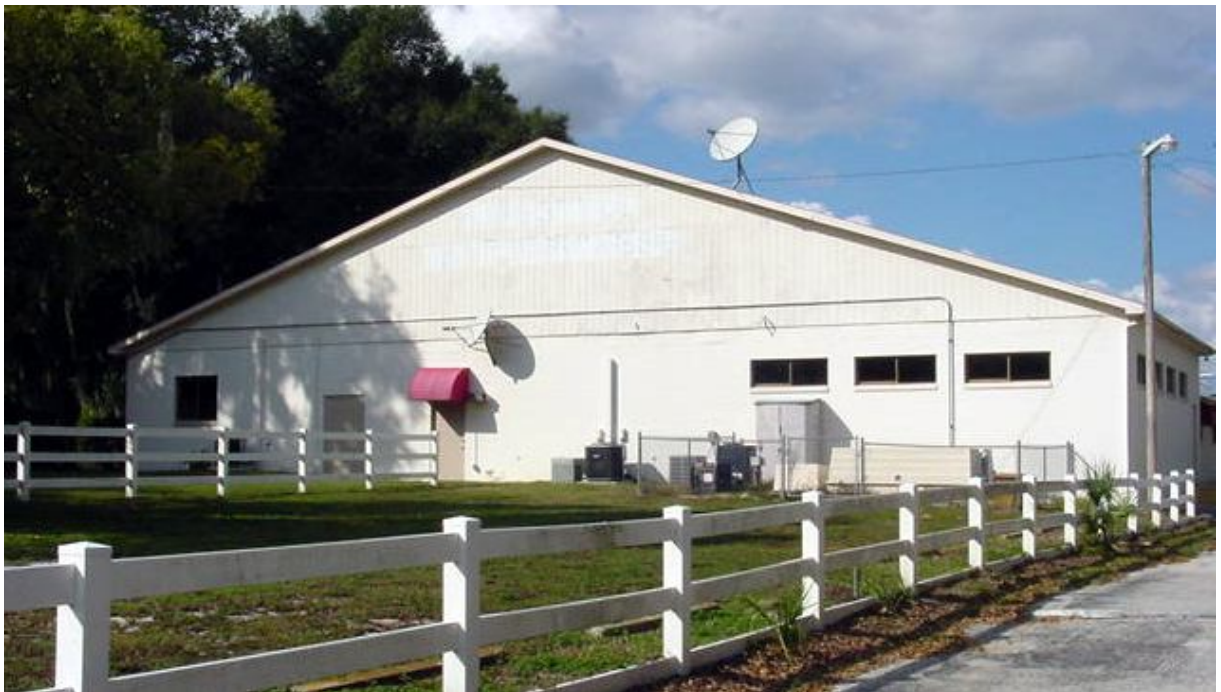
VIEW OF SOUTH SIDE OF SUBJECT BUILDING & GRASS PARKING AREA
