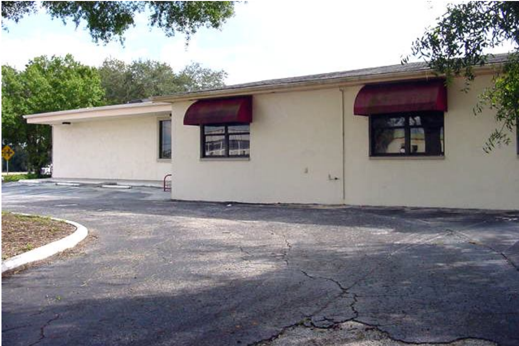
VIEW OF NORTH SIDE OF SUBJECT BUILDING AND CIRCULAR DRIVE
