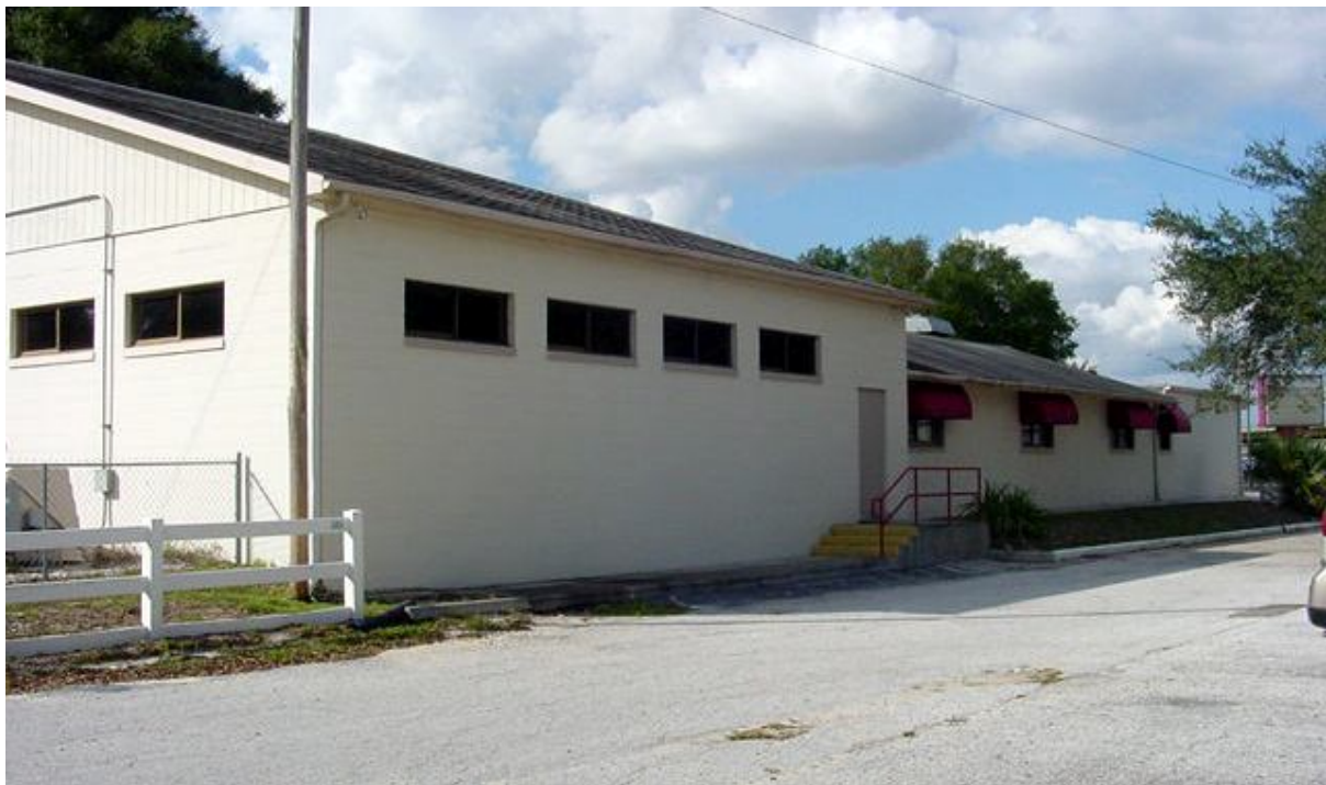
VIEW OF EAST SIDE OF SUBJECT BUILDING
