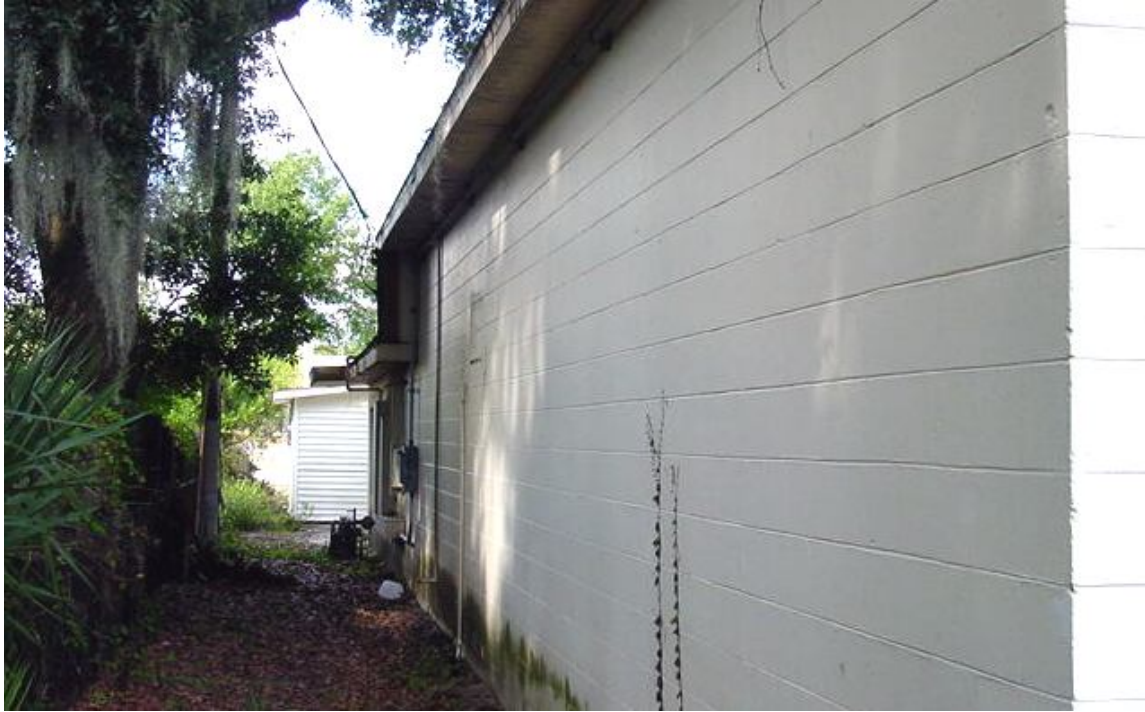
VIEW OF WEST SIDE OF SUBJECT BUILDING
