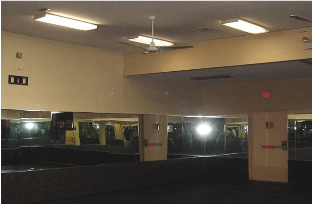
VIEW OF INTERIOR OF SOUTHWEST AREA OF SUBJECT BUILDING
