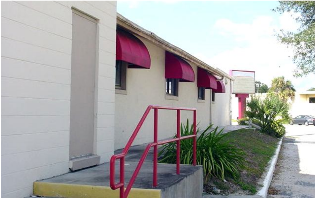
CLOSE-UP VIEW OF EAST SIDE OF SUBJECT BUILDING
